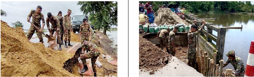
Picture 4: Repair and Reconstruction of Roads and Bridges by Army
