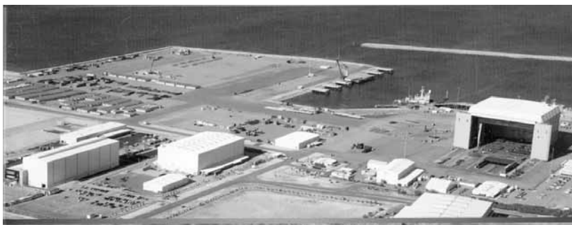
Figure 11 : View of a Common User Facility (AMC)
